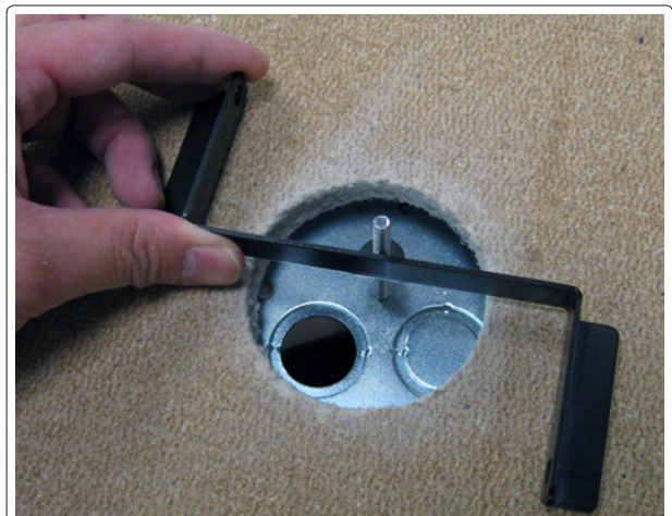
2b Attach the Z bracket loosely to the ceiling tile and the back plate.
