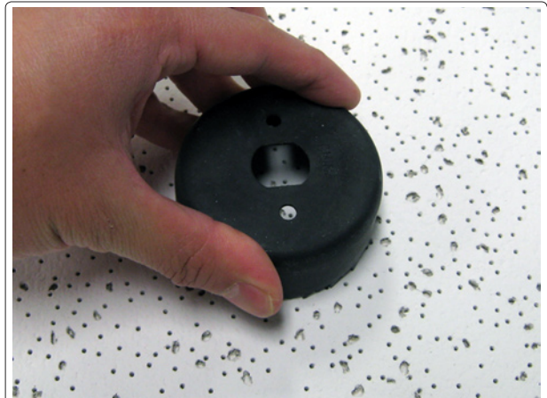
1b Cut a hole in the ceiling tile.
