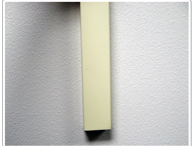
① Install the raceway (if needed).
