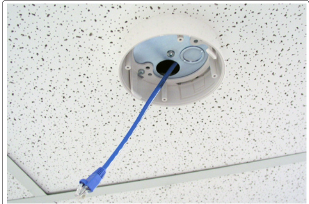
①a Pull the cable(s).
