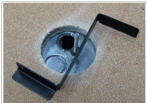
2d Secure the back plate to the ceiling tile and the Z bracket.
