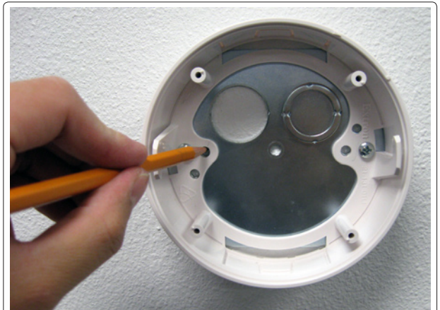
② Mark mounting screw locations in the surface.
