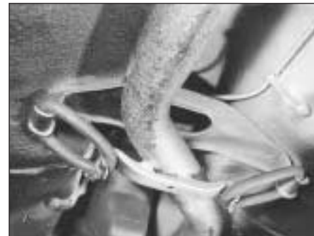
19.7A Exhaust pipe support rings
