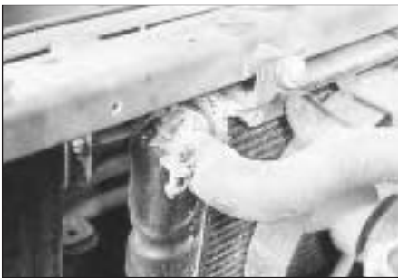
Leaking antifreeze often leaves a crystalline deposit like this.
