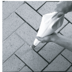
Figure 16 - Grouting Brick
