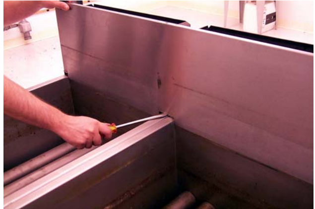
Removing flue cap.
