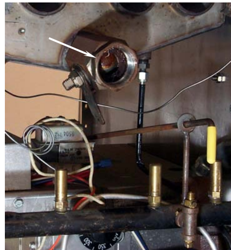
Ball retainer nut (arrow) on drain valve.
