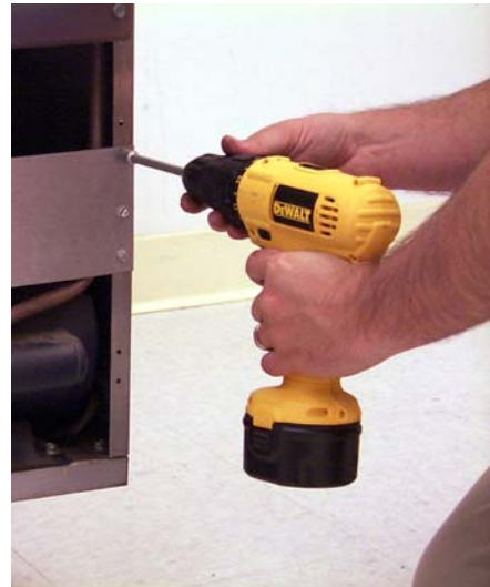
Removing gas manifold shield.
