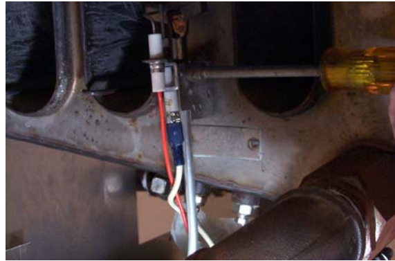
Removing electronic/standing pilot assembly.
