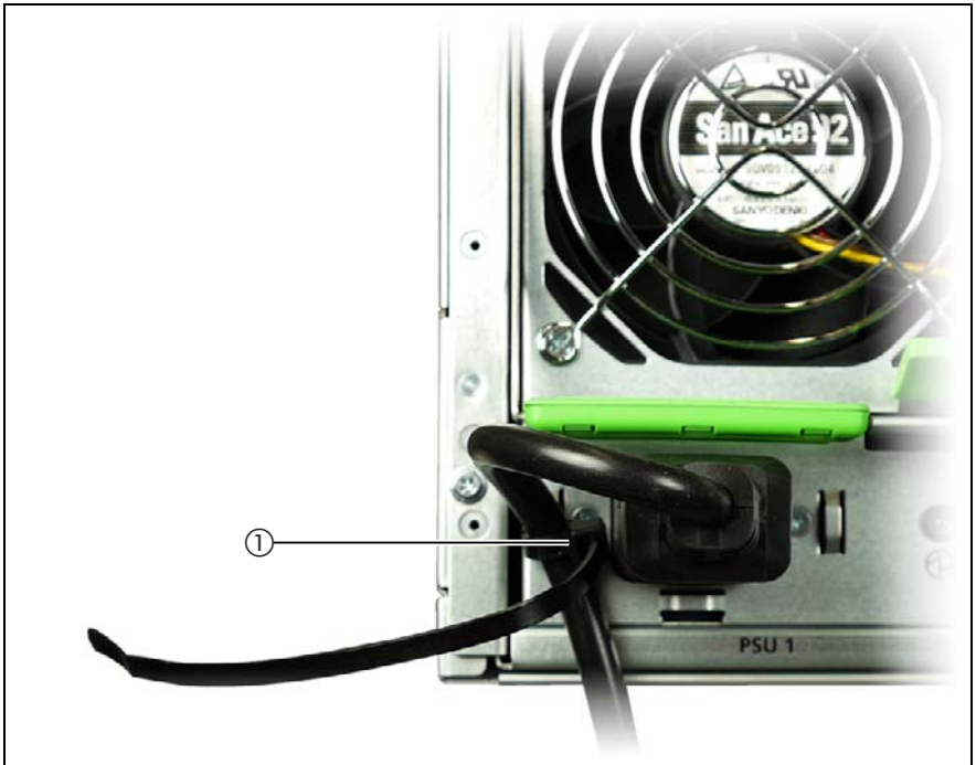
Figure 10: Using cable ties
