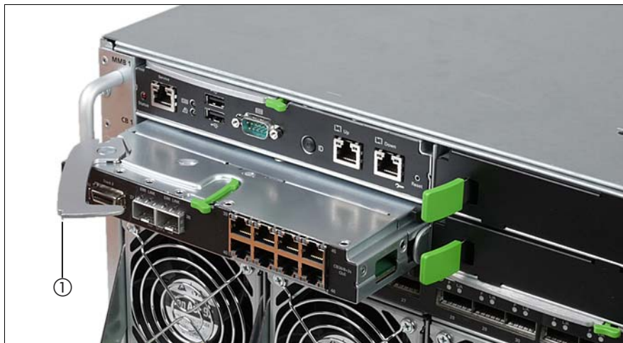
Figure 37: Installing a connection blade
