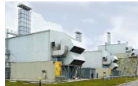
Blue Stream Pipeline Project from Turkey to Russia PGT25 - BCL406/b
