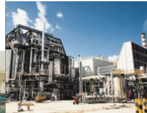
Livorno - Italy MS9001 Turbogenerator units for Refinery plant
