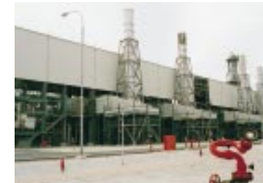
Ras Laffan Mesaieed - Qatar MS5002 Turbo units for LNG and Ammonia Synthesis
