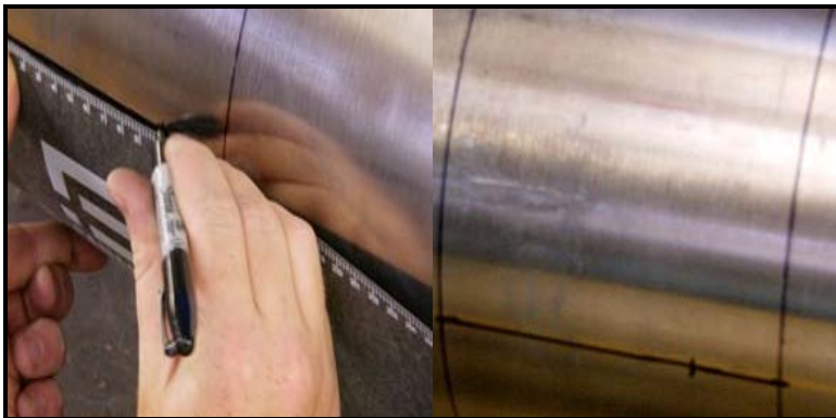
Figure 3-15: Marking the 9 o'Clock Position
