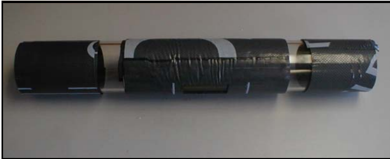
Figure 3-26: Completed DMP-1 Installation
