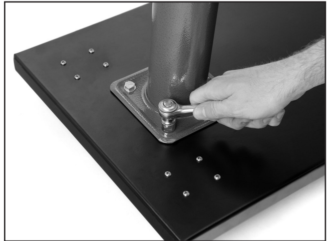
Figure 6. Installing collector support.
