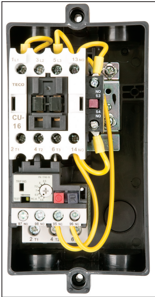
Figure 1. Model G4571 magnetic switch.
