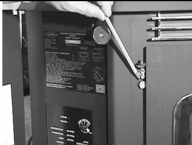
Fig.15: Draft Meter bolt hole location
