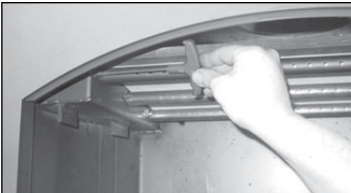
Figure 32.2 Removing Manifold Tube
