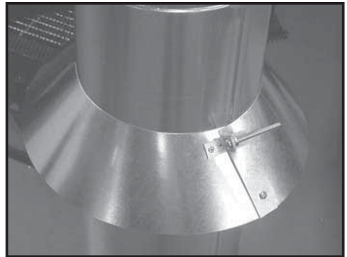
Figure 8.17 Assembling the Storm Collar Around the Pipe
