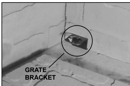
Figure 4.16 Sliding Bottom Refractory Towards Back of Fireplace
