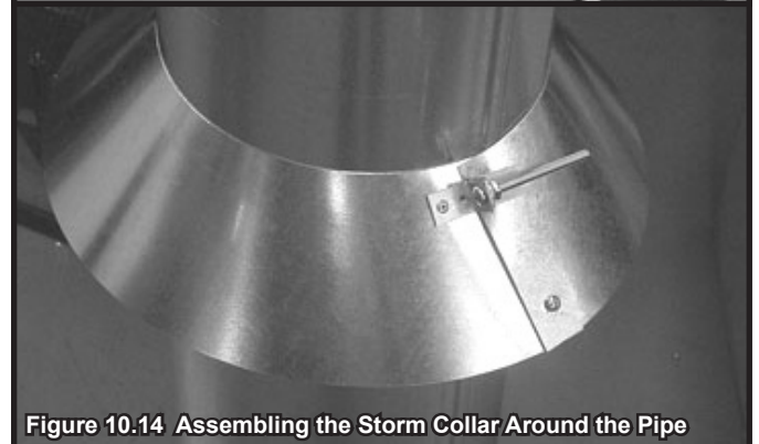
Figure 10.13 Assembling the Storm Collar
