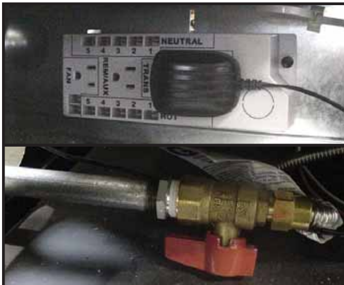
Figure 13.5 Preparation to Install Splatter Guard
