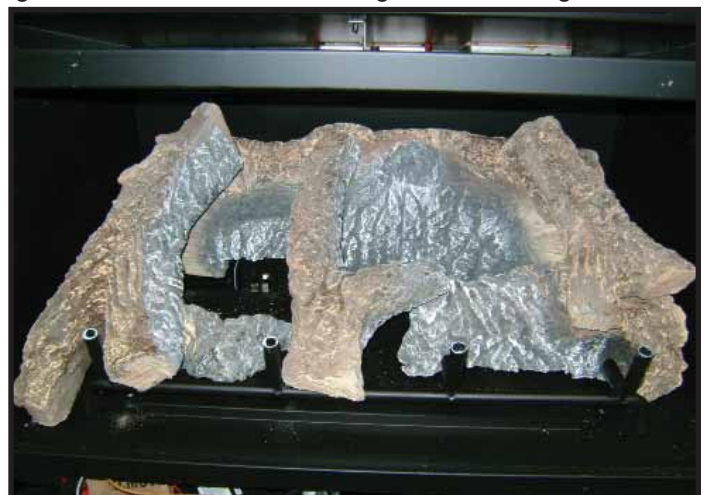
Figure 10. Log Set Installed
