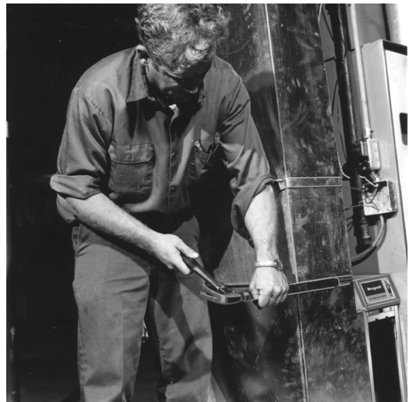
Fig. 25. Complete the duct installation.
