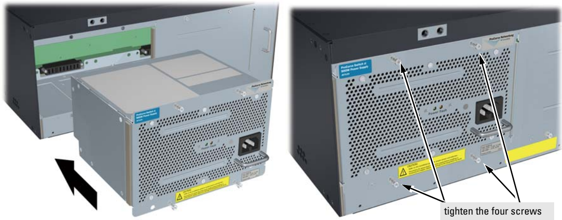
Figure 4-2. Power Supply Installation
